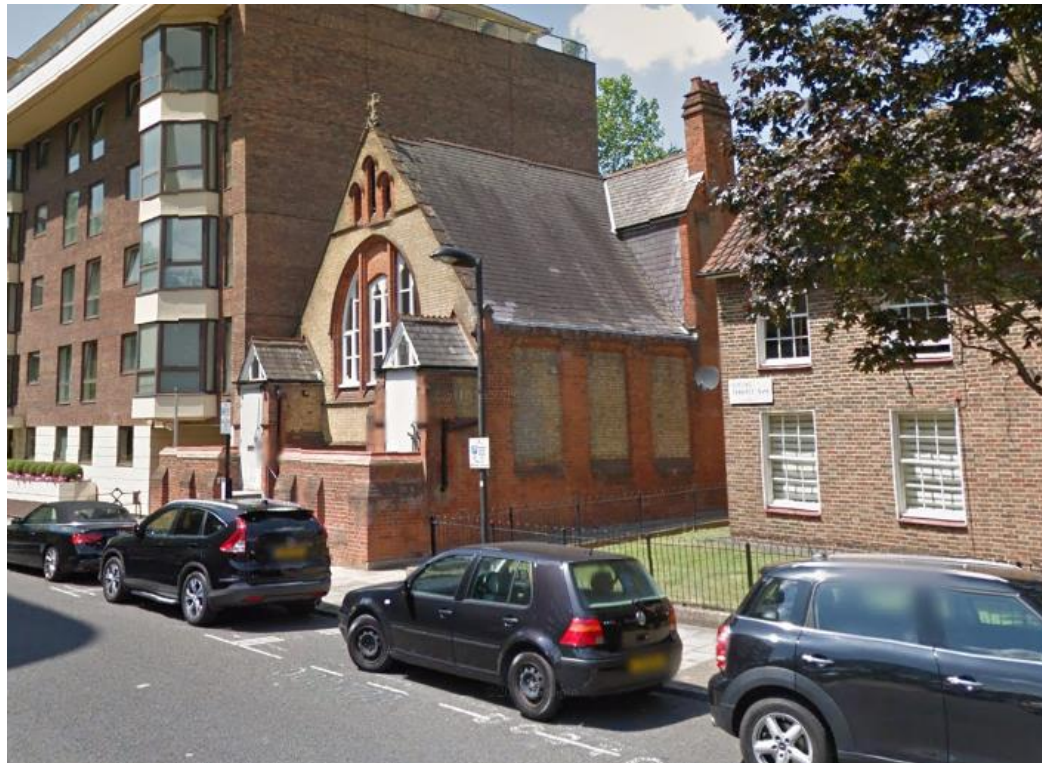
Site frontage and first floor
